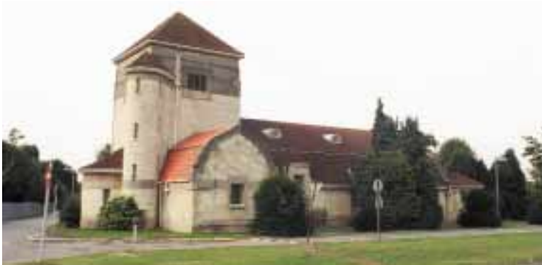
Runwell Mental Hospital, Chapel Exterior, 1937. Catalogue no. A2/A3 Photo: Derek Banham
